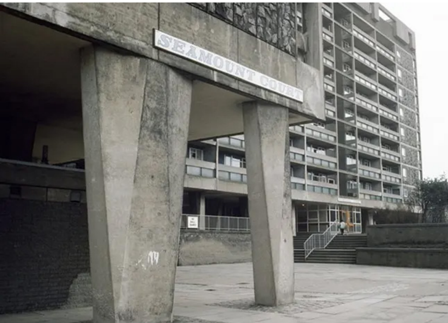
Seamont Court Apartment Block - Aberdeen, Scotland
