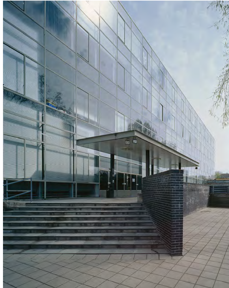
1. Flat full-glazed curtain wall, photo Ton Roelofsma (1967)
