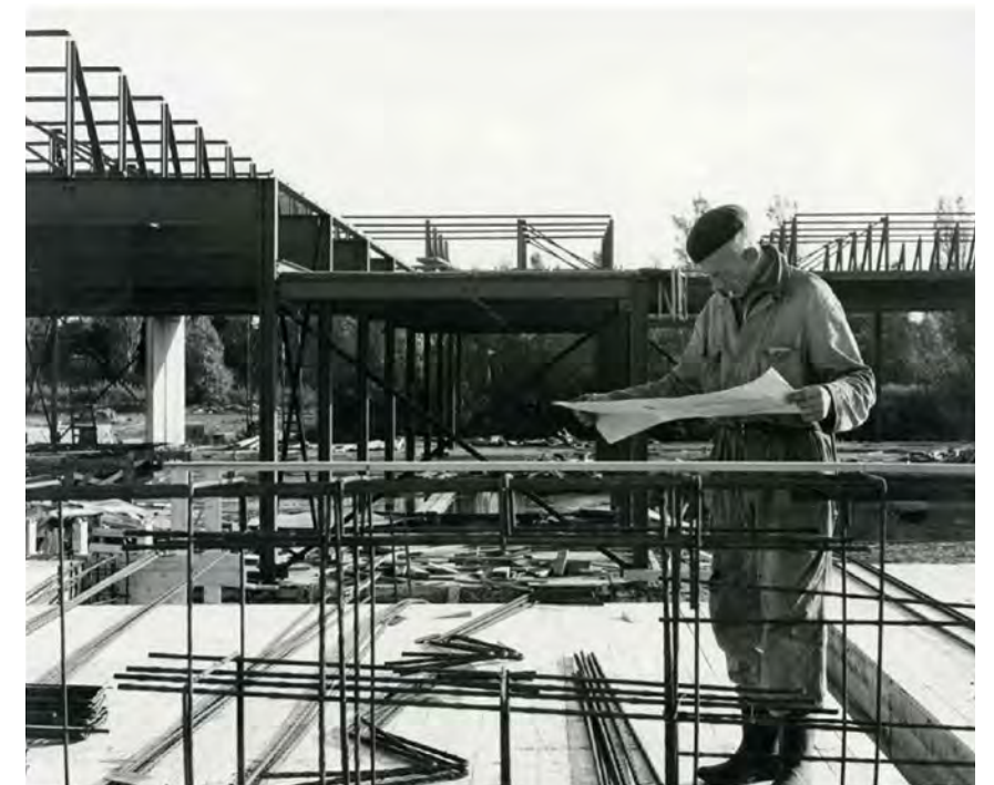
10. Construction of the steel structure of the workshops, 1964-1966, GRA
