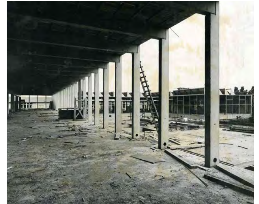
9. Construction of the concrete structure of the main volume, 1964-1966, GRA
