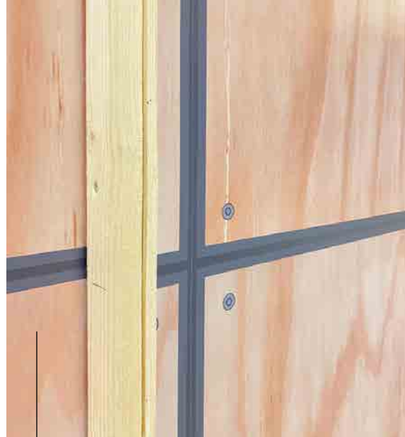
Fig. 16b Detail of the wooden wall at Almere Centrum.
